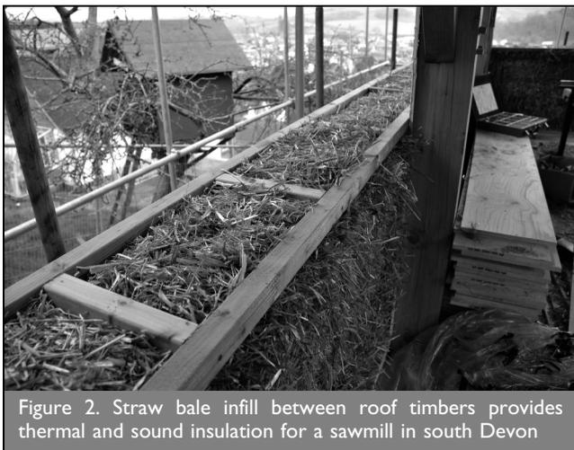
Figure 2. Straw bale infill between roof timbers provides thermal and sound insulation for a sawmill in south Devon
